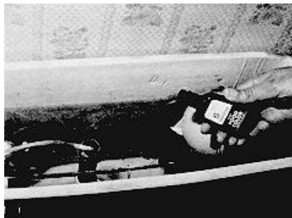
Figure 7a. Place food coloring in toilet tank.
