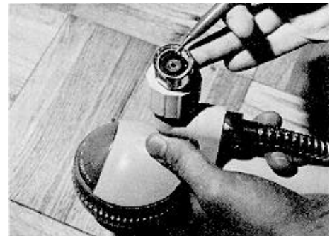
Figure 5b. Flow restrictor in place.
